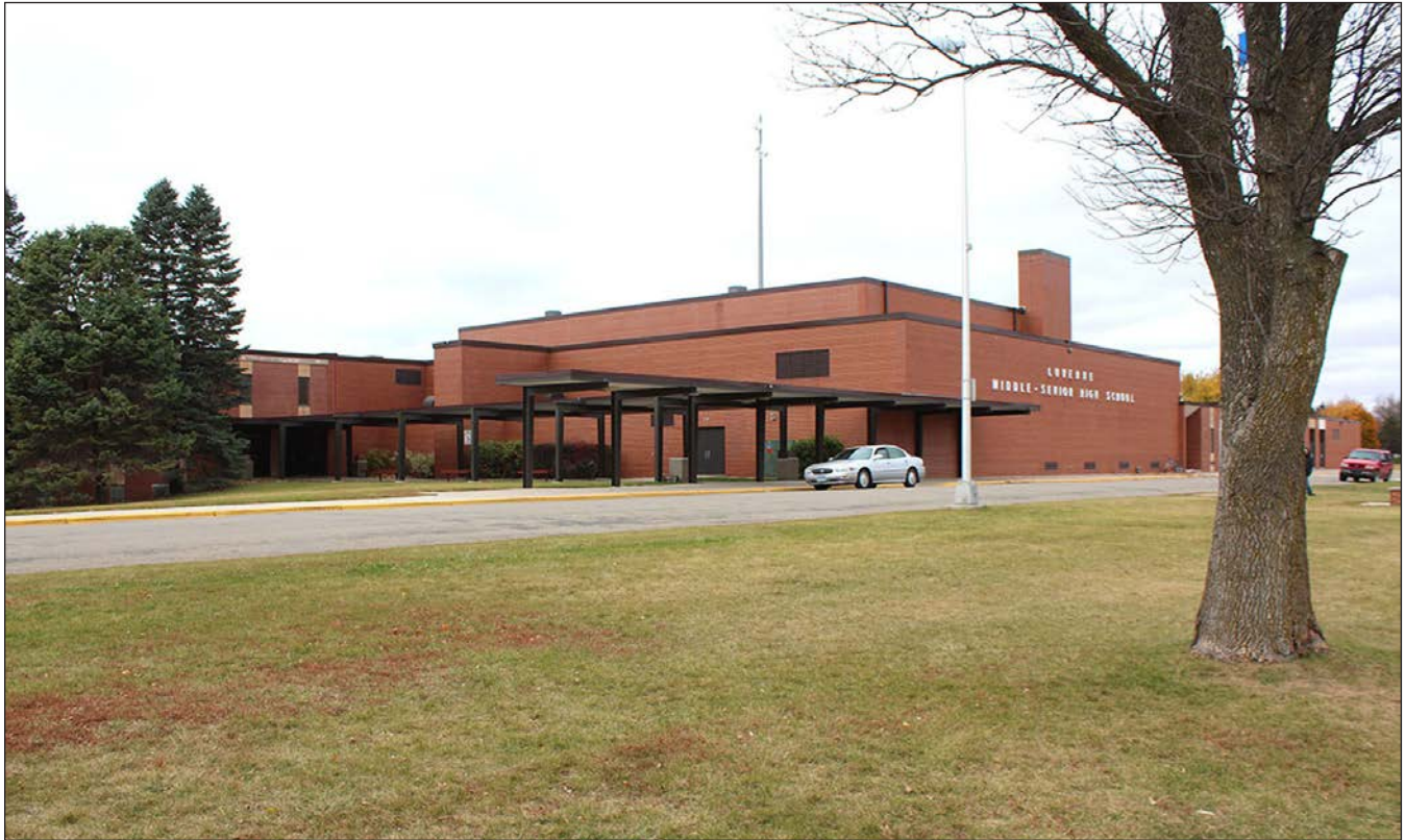
The east side main entrance of Luverne High School Middle School looks mostly the same as it did when it was first constructed in the 1950s. After the new project is complete, the main entrance will be on the south side of the complex.
